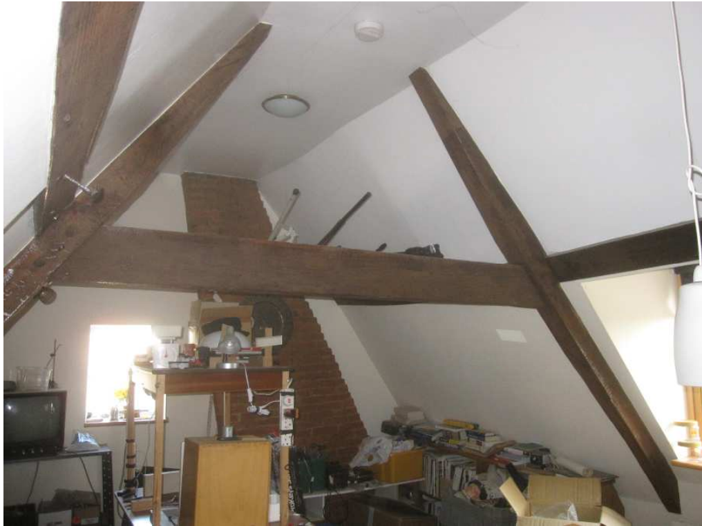
The eastern A-frame truss to the main range
