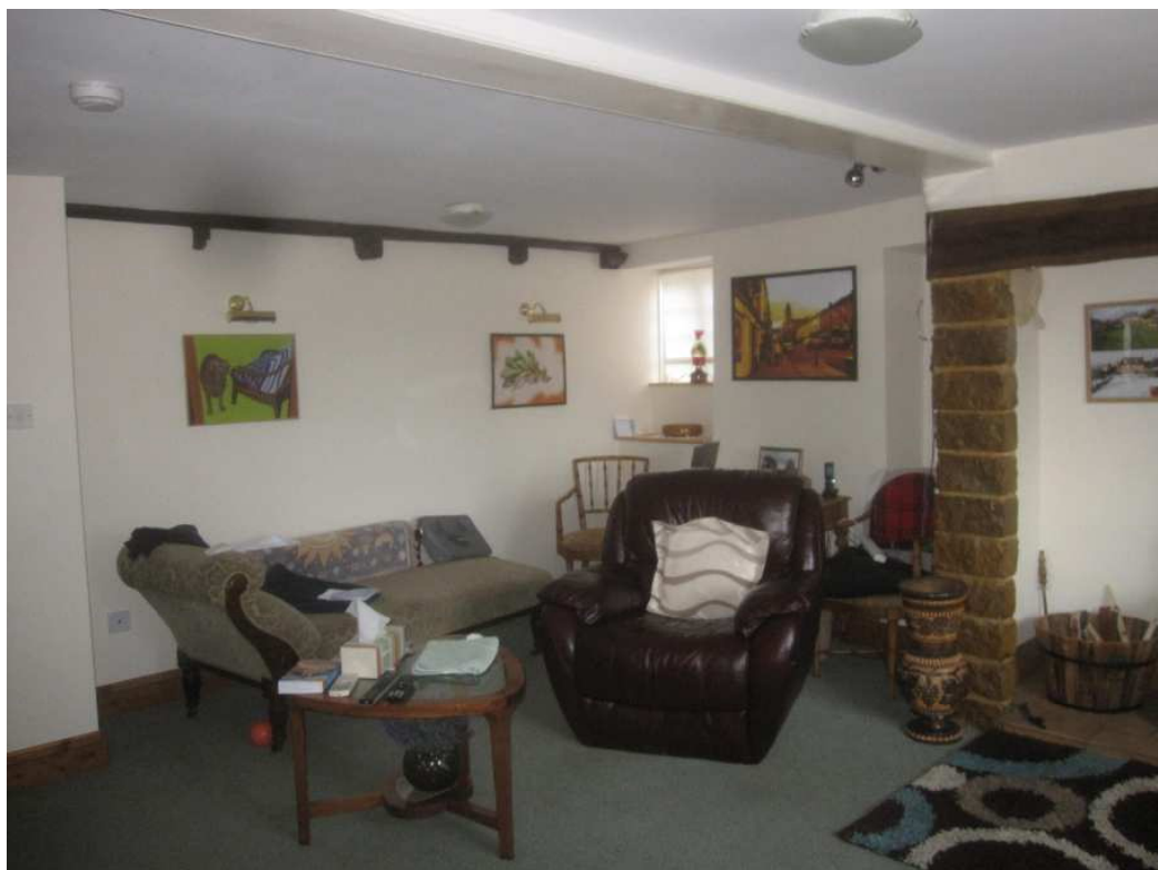
The east room of the main range, with corbelled timber plate to north wall
